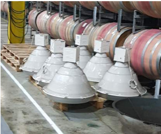
Removal of old HID lighting
